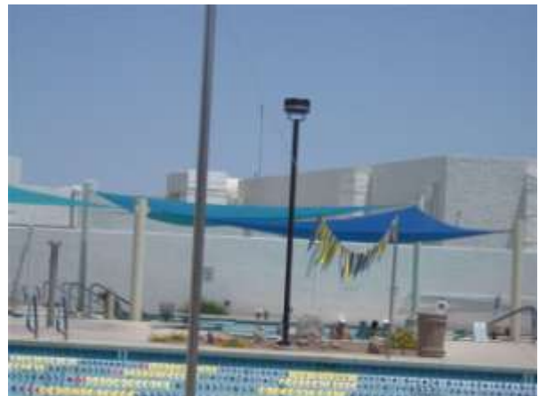
Bell pool parking lot lights
